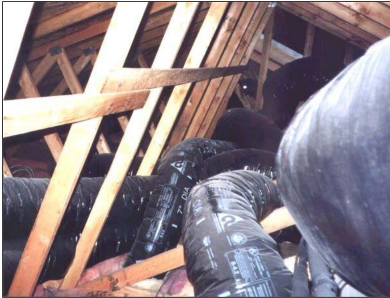
Figure 1. Ducts in an Unconditioned, Vented Attic
